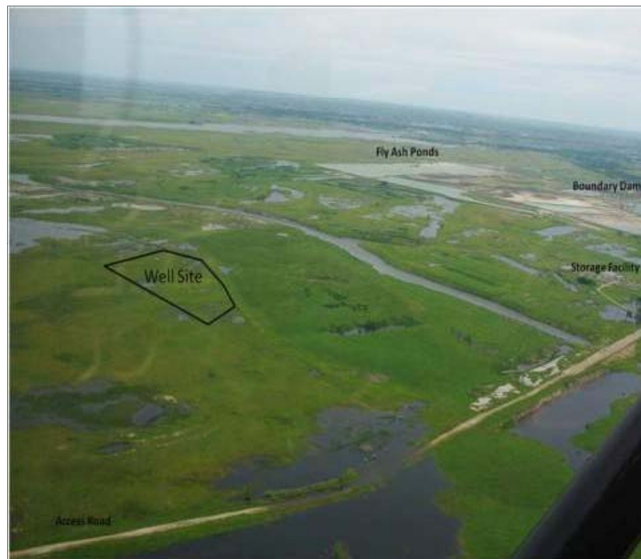
Well location remains largely free of water during the 1:500 year flood in Saskatchewan 2011
