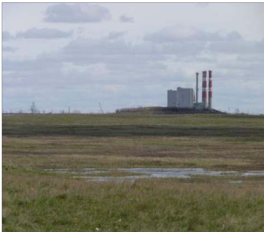
Ground level view towards Boundary Dam Power Station
