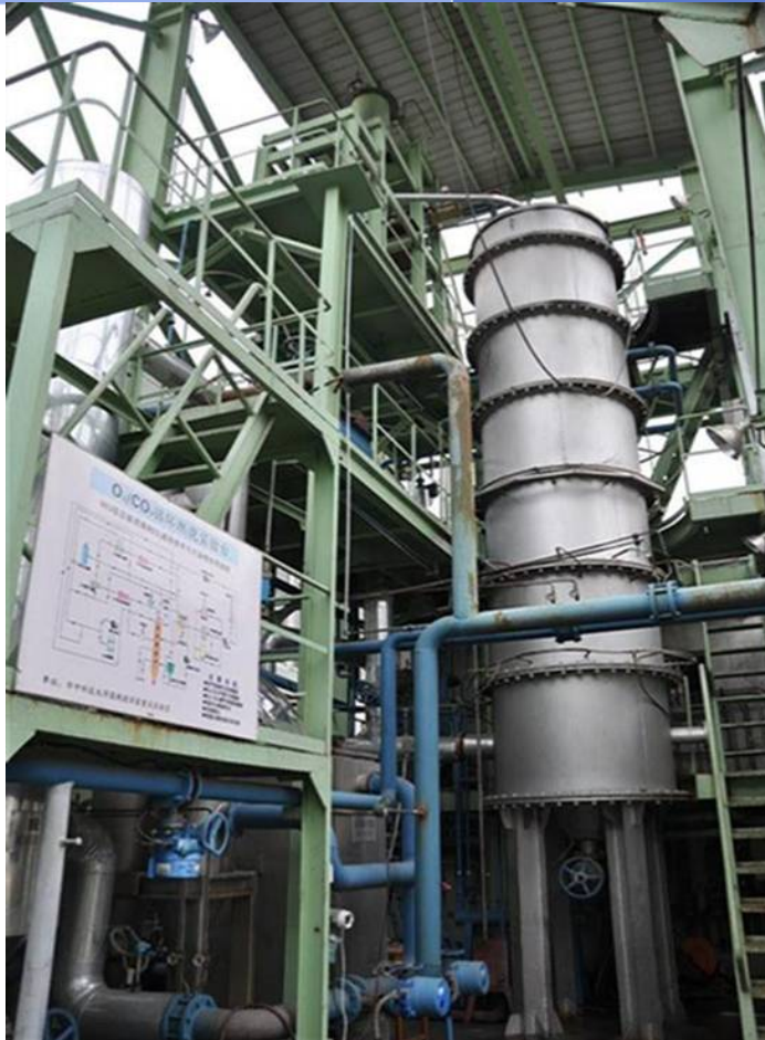
Existing 400kWt Oxy-fuel recycle combustion facility
