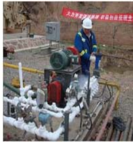
CUCBM CO 2 -ECBM Well Site
