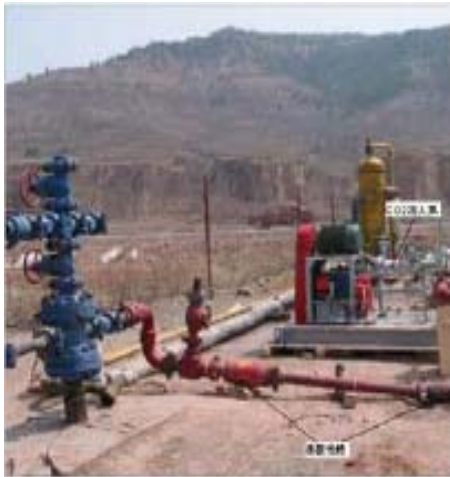
CUCBM CO 2 -ECBM Well Site
