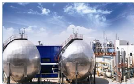
提纯、压缩 CO 2 纯度: 99.99% Purification and Compress (CO 2 purity: 99.99%)
