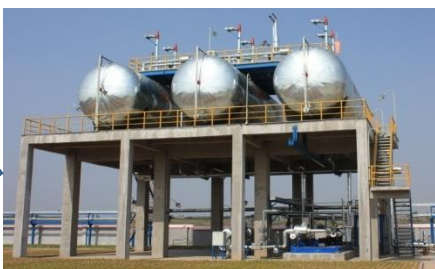
缓冲罐区 加压、增温, 泵注 Buffer tanks (compression, warmming and pump in)
