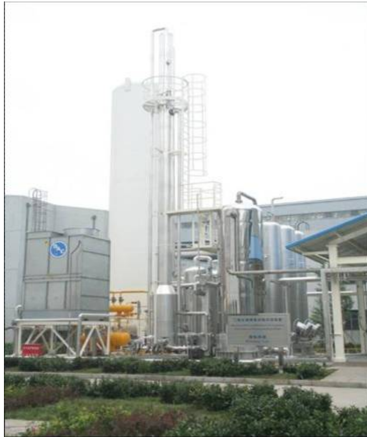
Huaneng Beijing Gaobeidian Thermal Power Plant, start operation in 2008, CO 2 used in food industry
