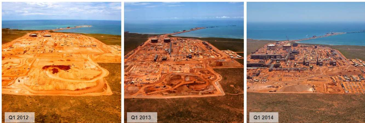
Time-lapse images of the LNG plant on Barrow Island
